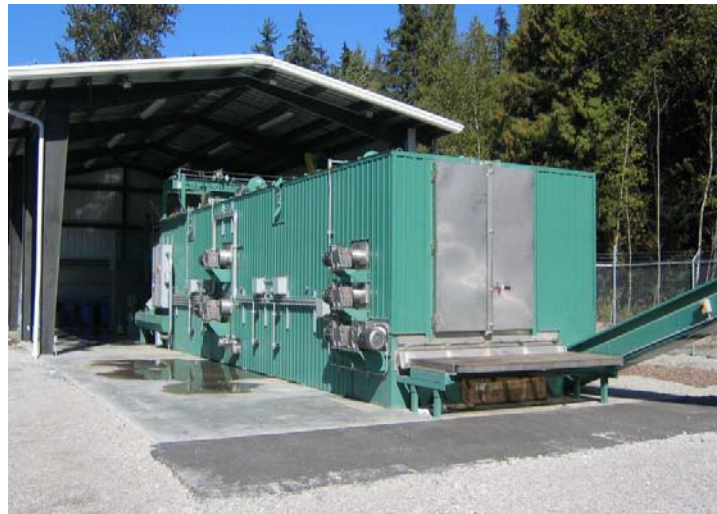
Figure A 3. UBC In-Vessel Composter
